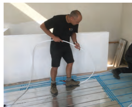
Insulated floor retrofitted into a home
